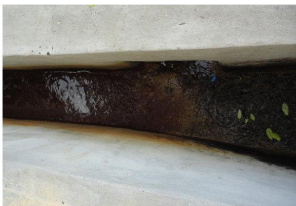
13. Acid started depositing due to final slope difference.
